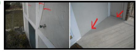
Attention Needed - The columns on the front porch are not sealed to the slab. Sealant needed to prevent further moisture deterioration.
